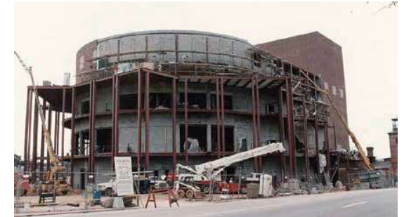
Peace Center under construction. Source: Greenville Journal, 2020
